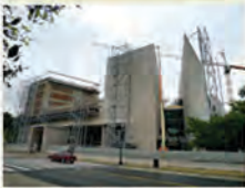
The National Gallery of Art East Building, with ongoing façade repair
